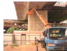
Installation of prism on the bypass
