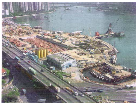
Tsuen Wan Station under construction
