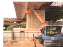
Installation of prism on the bypass
