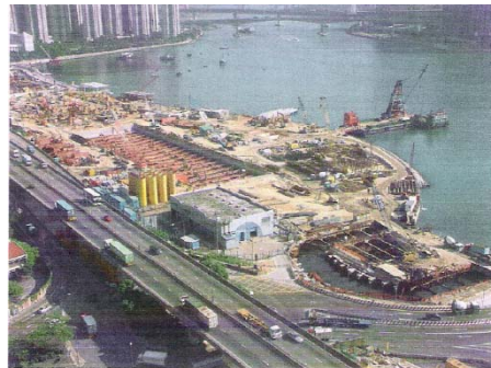
Tsuen Wan Station under construction
